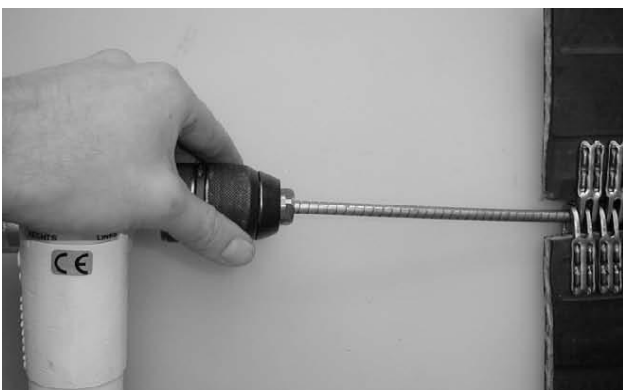
13. ...pull the tool approx. 30cm back, clamp the chuck and operate again.
